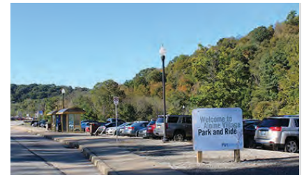
Park and Ride Facility in Alpine Village, PA
