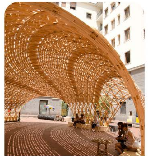
C9 Performance pavilion/ outdoor classroom
