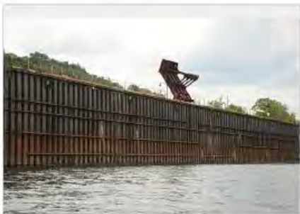
Giant Bulkhead Wall
