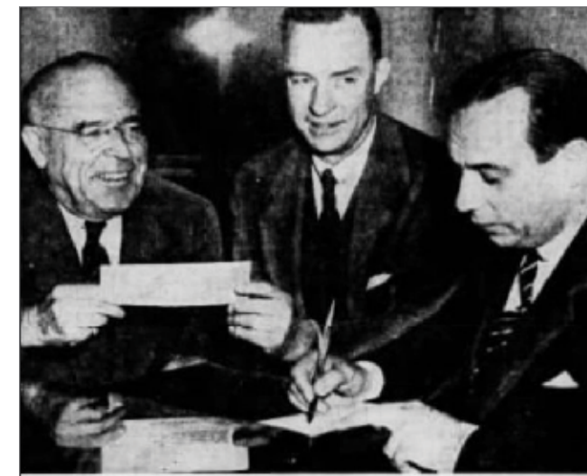
A CHECK FOR $100,000 is turned over to the City to vacate streets in an area between Second Avenue and the Monongahela River. Jones & Laughlin Steel Corp. will install a battery of coke ovens there. Left to right are Mayor David Lawrence, President C. L. Austin of J. & L., and Adolph Schmidt, vice-chairman of the Urban Redevelopment League.
