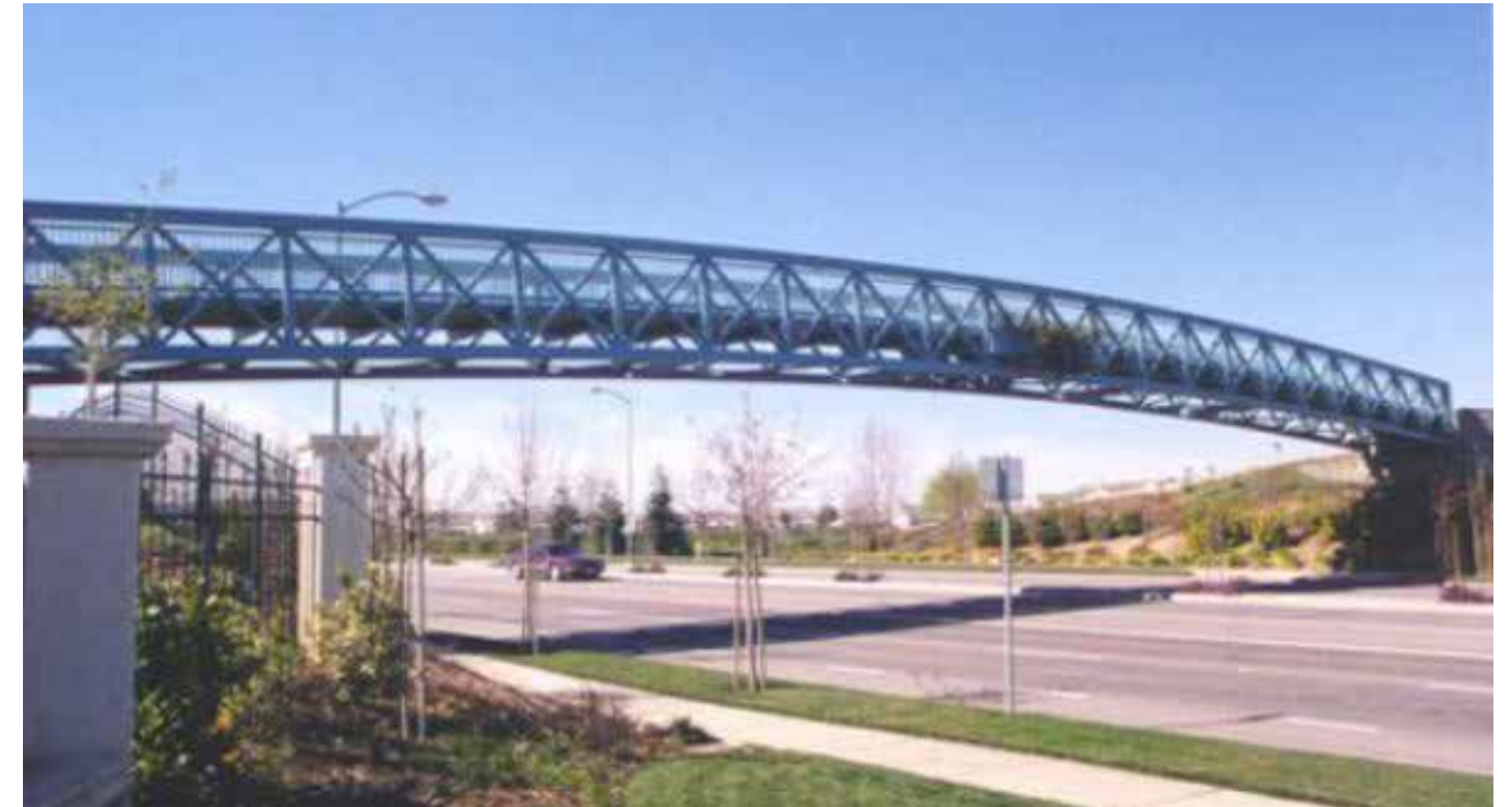
EXAMPLE OF A TRUSS BRIDGE
