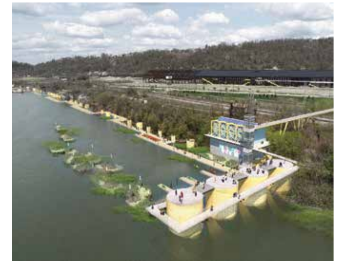
FUTURE VISION AT THE PUMP HOUSE
