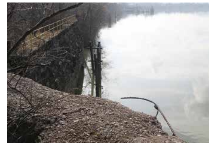
SITE PHOTO ALONG THE RIVER'S EDGE
