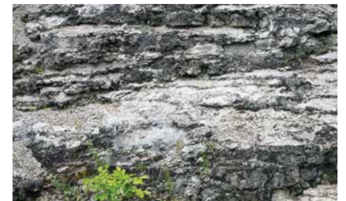
SITE PHOTO OF FLY ASH DETAIL
