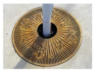
New installations also include six tree grates designed by Pittsburgh-based artist Carin Mincemoyer and fabricated by Technique Architectural Products. Constructed of raw steel that will be allowed to rust naturally on site, the tree grates feature images of the leaves and nuts of the hazel tree, a species that once grew in abundance along the banks of the Monongahela and for which the neighborhood is
